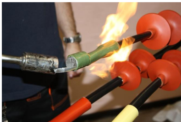
Fig. Installation heatshrinkable cuffs, casings and insulating cuffs on electric cables.
